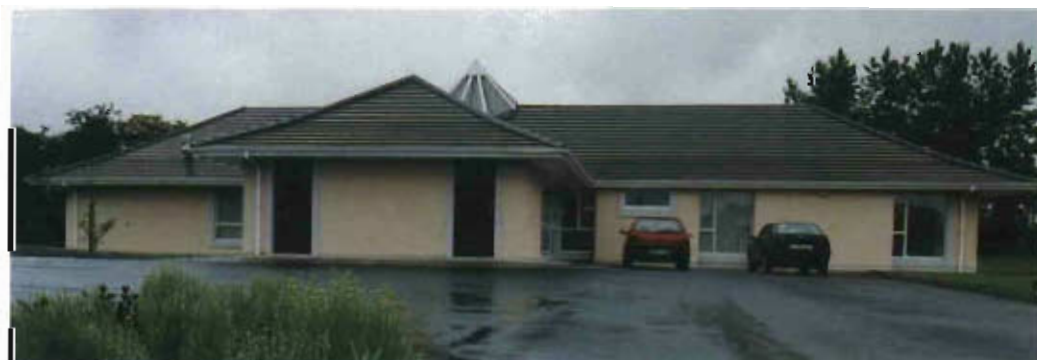
New Family Resource Centre at Commons Road, Navan
