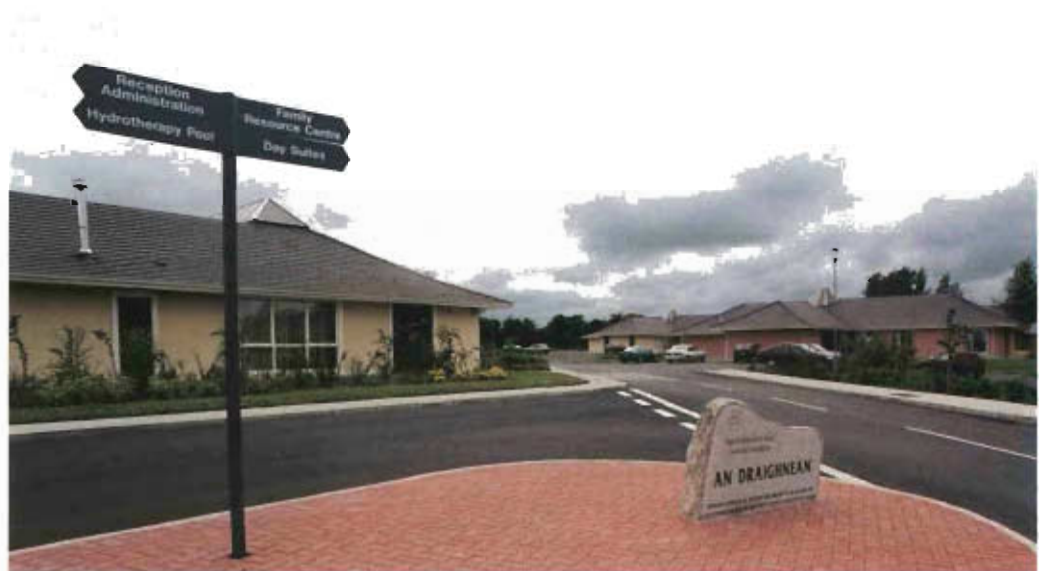
New facilities at An Draighneán, Navan which includes residential day-care and respite facilities for people with disabilities.
